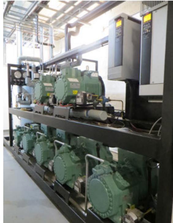
Electricity for refrigeration makes up 50% of the total energy consumption of the store. Makro has an ambition to cut down this consumption year by year as part of their sustainability program. Another goal is to switch to natural refrigerants like CO2 to cut the carbon footprint.
